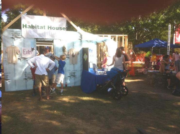
Entryway to this year's Habit for Humanity house under construction. Hammers were handed out to all those who willing to drive a nail.
